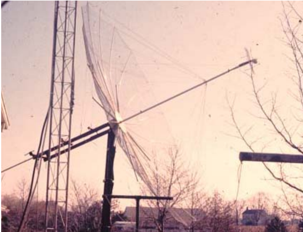
Figure 1. Twenty foot stress parabolic reflector used on 432 EME for many ears at K2UYH and later W3CCX.
