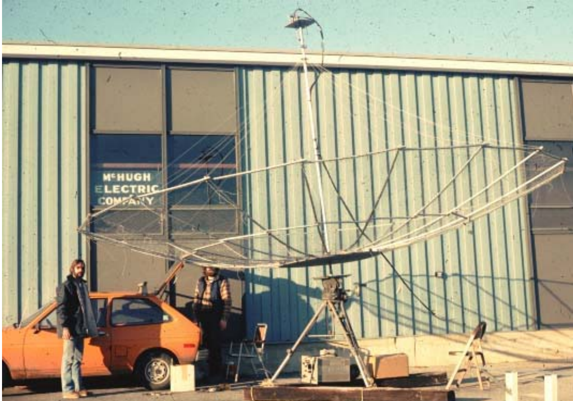
Figure 8. Portable 20 foot stress dish in DE. Carried on top of car.
