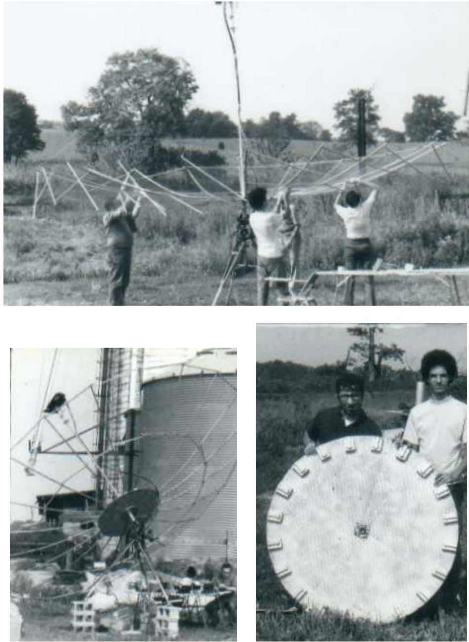
Figure 10. Portable 20' stress dish. a) Assembly, b) In operation, and c) Center hub.
